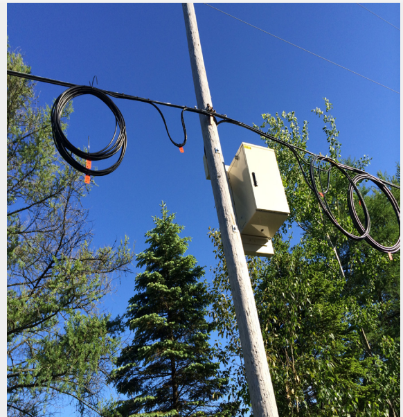
Bell Canada Optical splitter for FTTP deployment on Rang St-Dominique (corner of Ménard) between St-Lazare and St-Clet Québec. Rural farming area without DSL.
